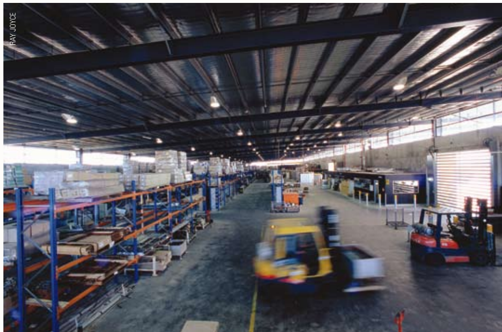
ABOVE: The iconic roof encloses 5,500m 2 of column-free space where forklifts and mobile cranes are used to move equipment, spare parts and electricity poles through storage and workshop facilities
